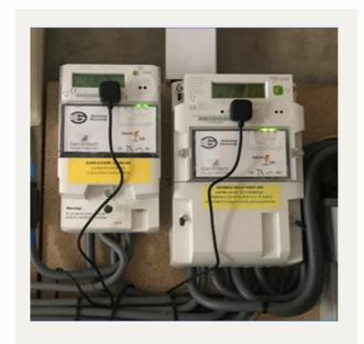
This image shows the Energy Monitor sensors fitted to a singlephase meter on the left, and a three-phase meter on the right
